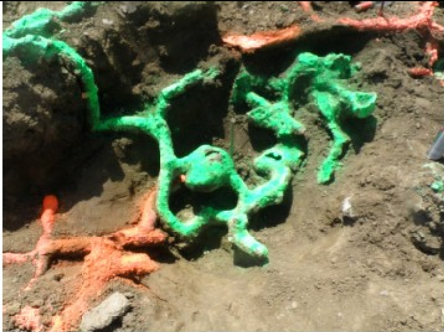
Photo 4A -29. Group of ground squirrel dens connected to smaller gopher holes, Clayey Levee.
