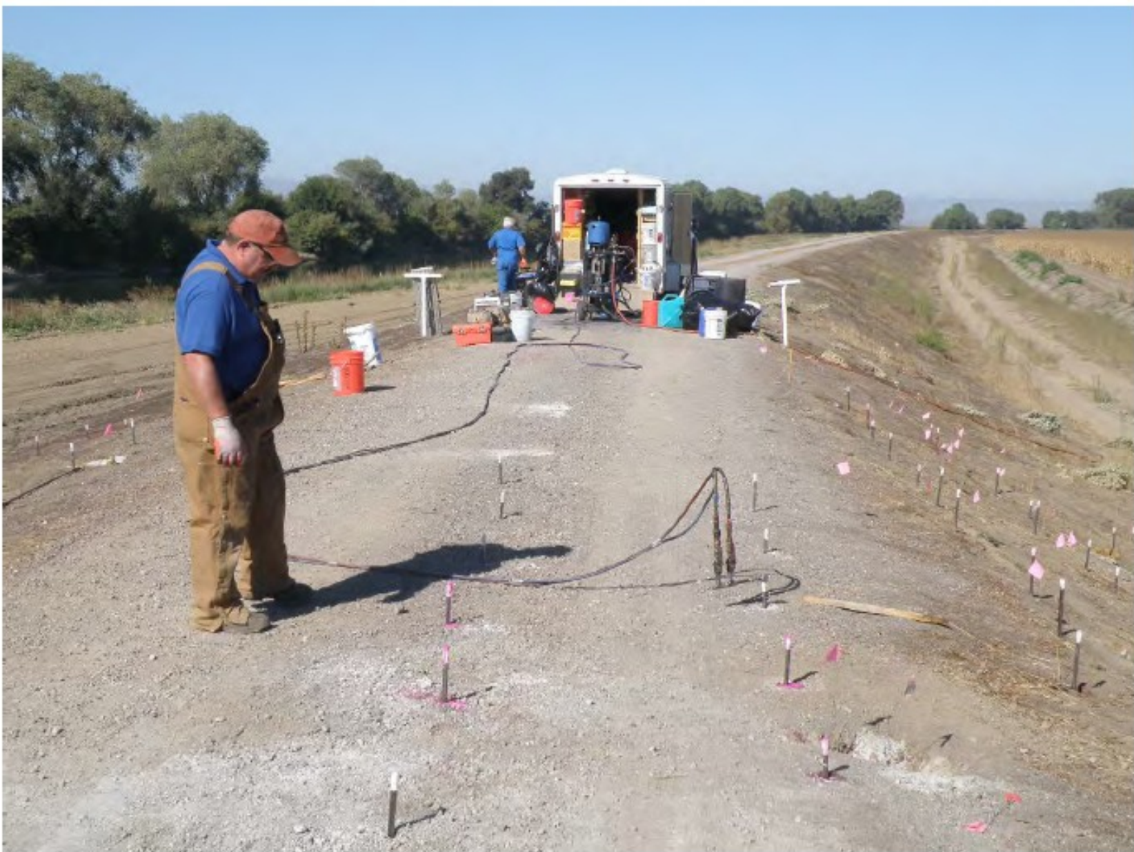
Figure 2-8. View of chemical grout injection procedure
